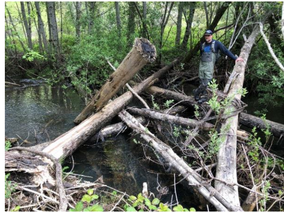
Example accelerated recruitment, cross-channel large wood structure from the Phase 1 project.
