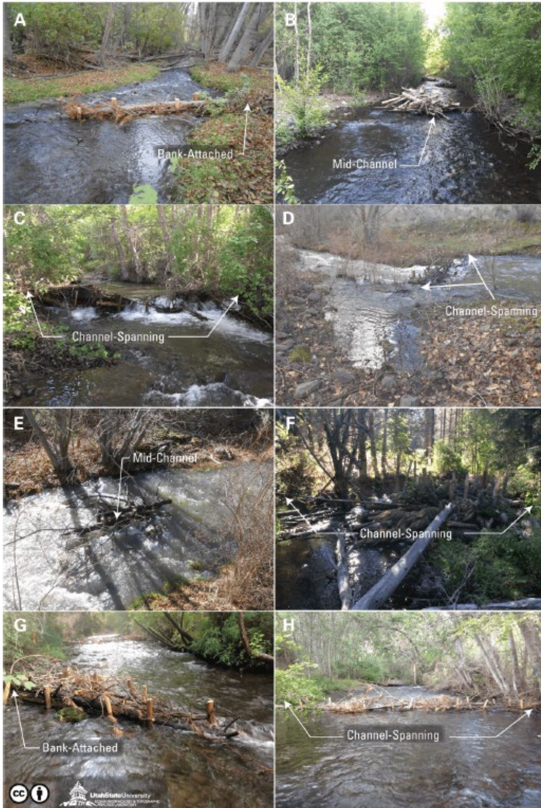
Figure 26. Examples of different types of PALS, designed to achieve specific objectives. PALS can be bank-attached, mid-channel or channel-spanning.
